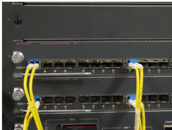
Figure 6: Some Examples of LASER Labels Found in the Verizon Network
